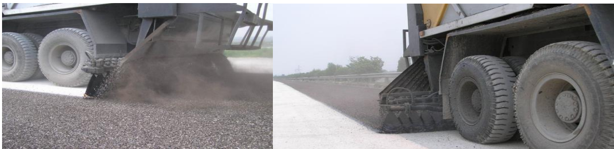
1.34-rasm. DAGANG SX5255TBS chipsilerida sirtga ishlov berish jarayoni
