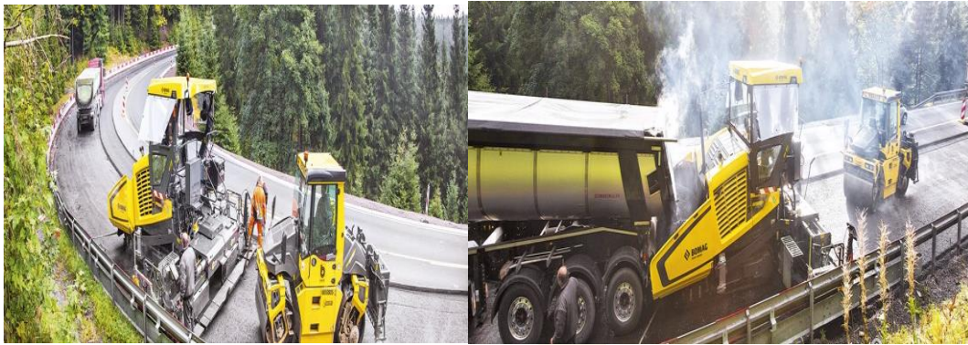
1.26-rasm. BOMAG kompaniyasining S500 markali asfaltyotqizgichi
