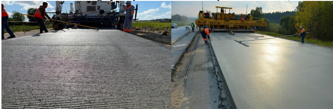
2.19-rasm. Yotqizilgan sementbeton qoplama yuzasini pardozi berish
