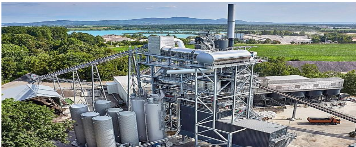
3.8-rasm. Benninghoven asfaltbeton qorishmalarini tayyorlash zavodi
