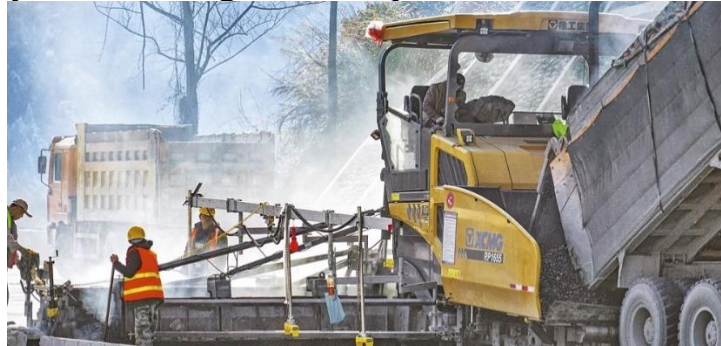
1.23-rasm. XCMG kompaniyasining RP1655 markali asfaltyotqizgichi
