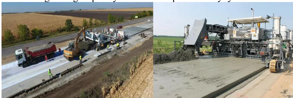
2.18-rasm. Beton qorishmasini yoyish
