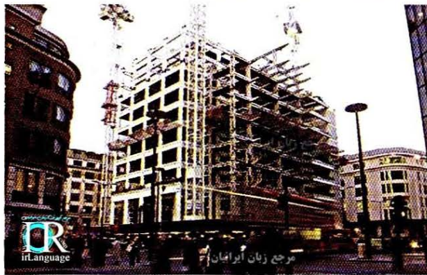
Steel beams make taller structures possible.
