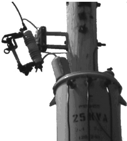
Figure 5-24 Distribution fuse.
