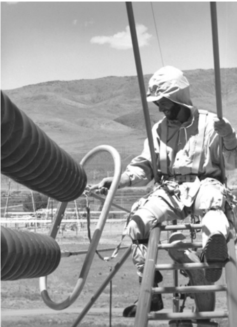
Figure 10-9 Bare hand live line maintenance.
