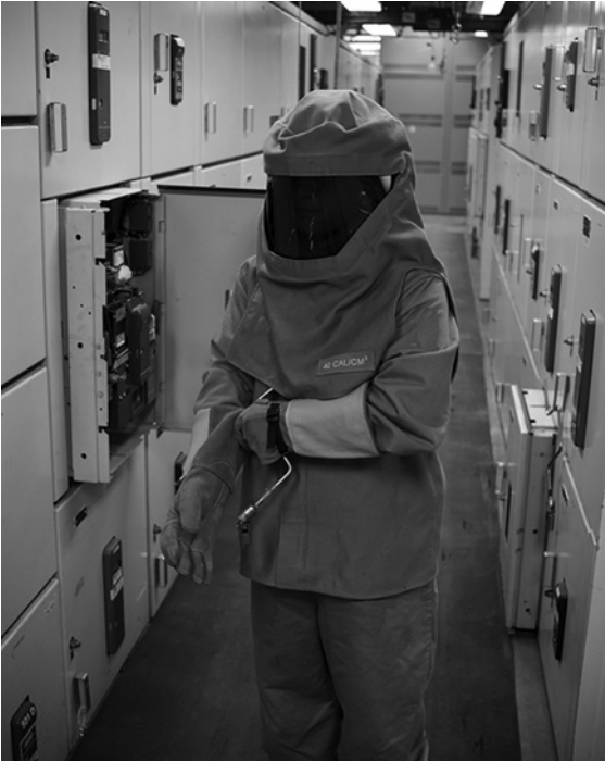
Figure 10-14 Arc-flash clothing. Reproduced with permission of from LSelectric.
