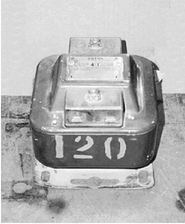
Figure 4-14 Low-voltage PT. Courtesy of Alliant Energy.
