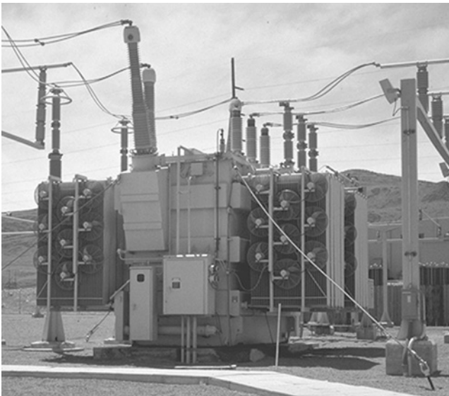
Figure 4-1 Step-down transformer.
