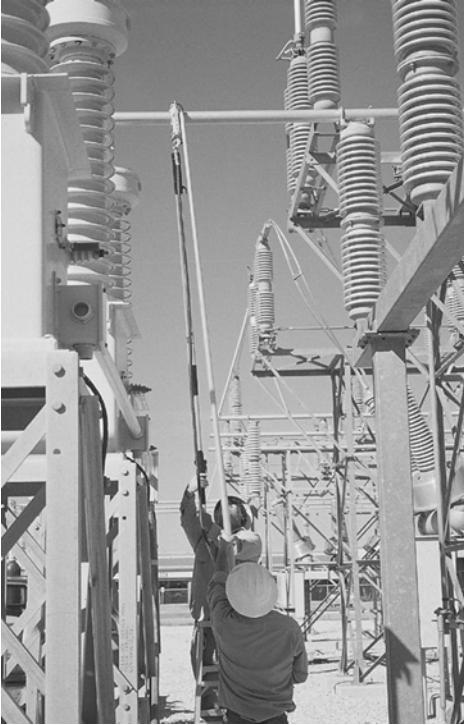
Figure 10-8 Live maintenance transmission lines.
