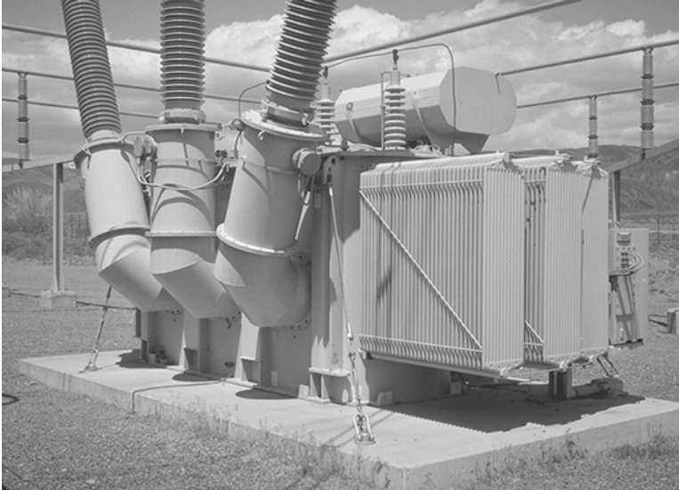
Figure 4-43 345 kV reactor.
