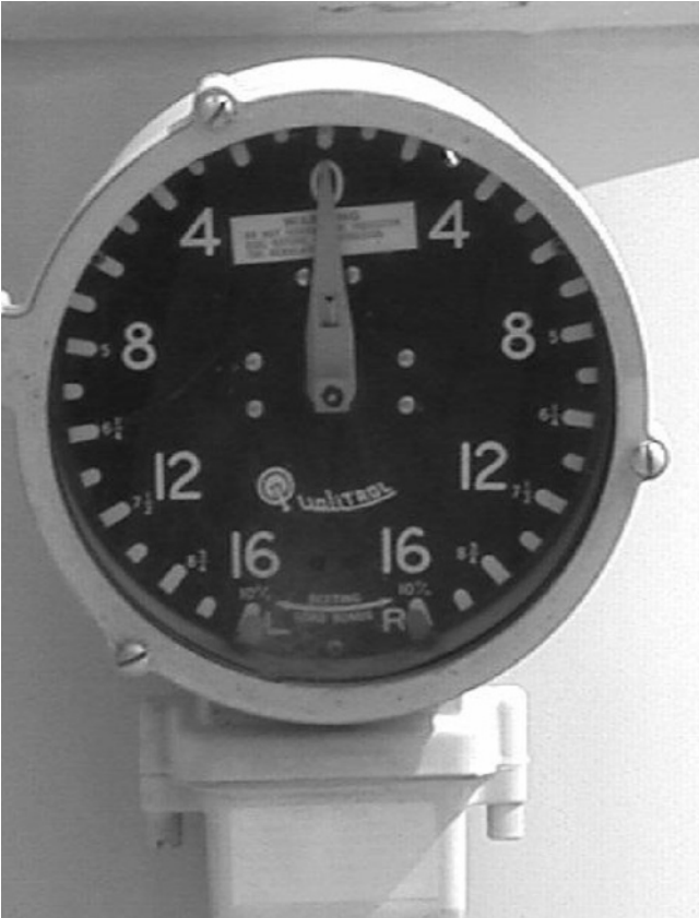
Figure 4-19 Regulator dial. Courtesy of Alliant Energy.
