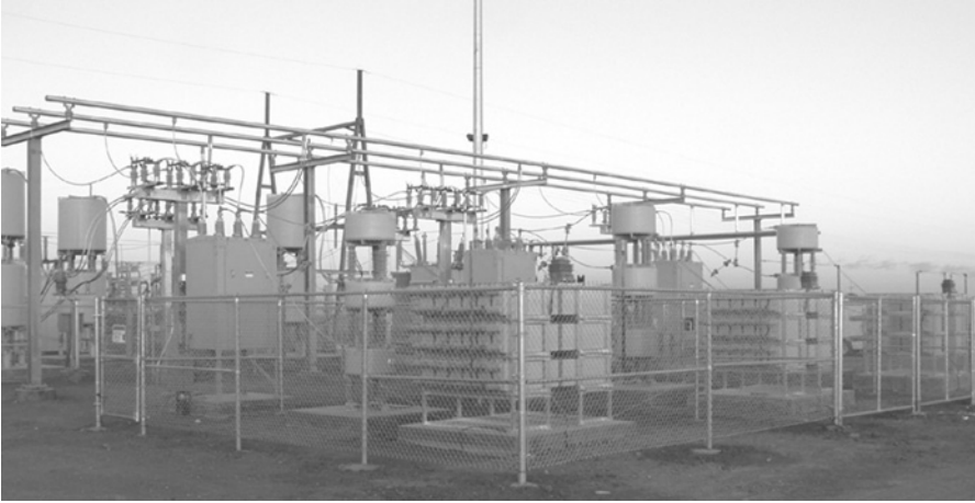
Figure 4-45 Static VAR compensator. Courtesy of Jeff Selman.
