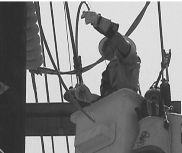
Figure 10-11 Live maintenance distribution. Courtesy of Alliant Energy.
