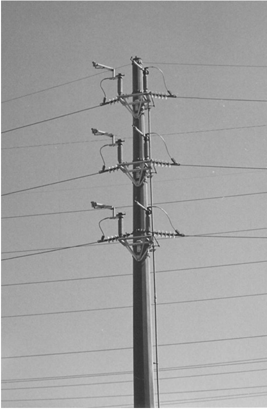
Figure 4-37 Line switch.
