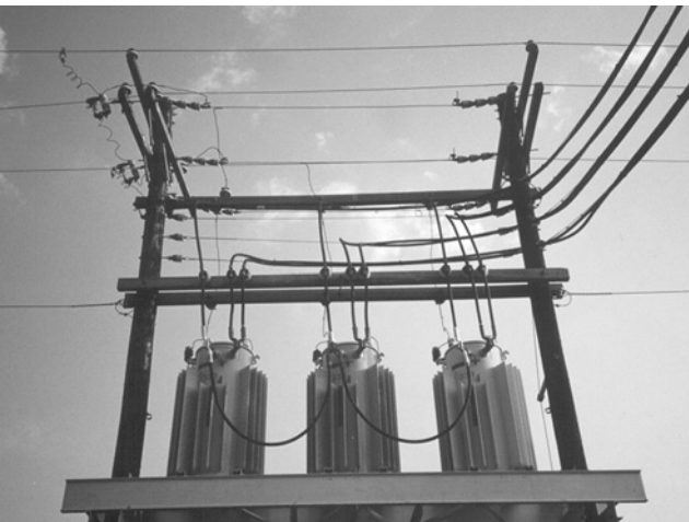
Figure 4-3 Transformer bank.
