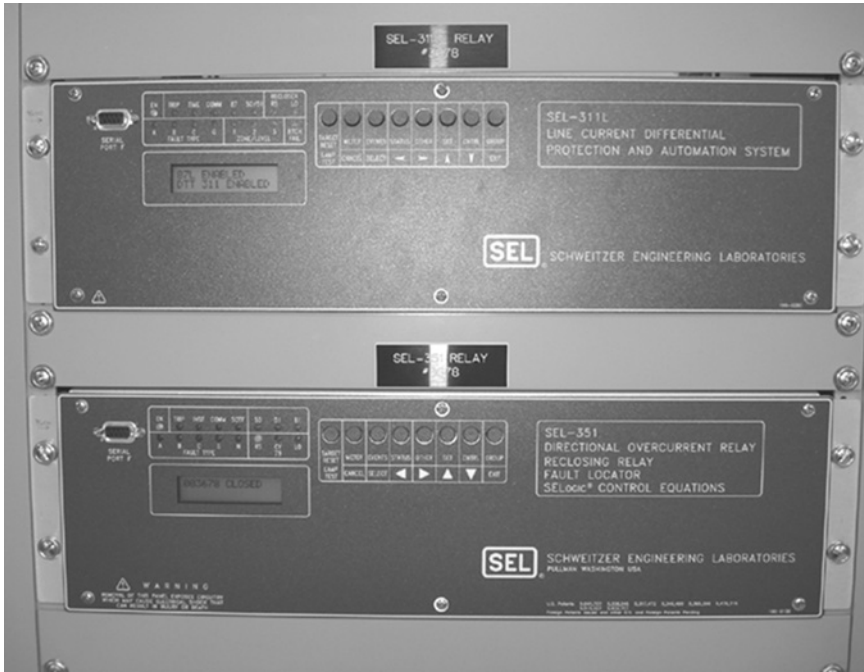
Figure 7-1 Solid-state relays.
