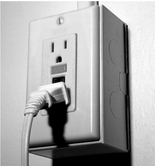
Figure 10-17 GFCI receptacle. Reproduced with permission of Photovault.
