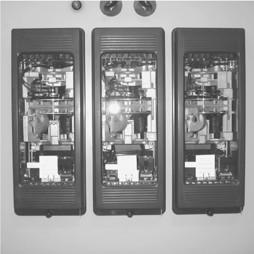
Figure 7-2 Electromechanical relays.
