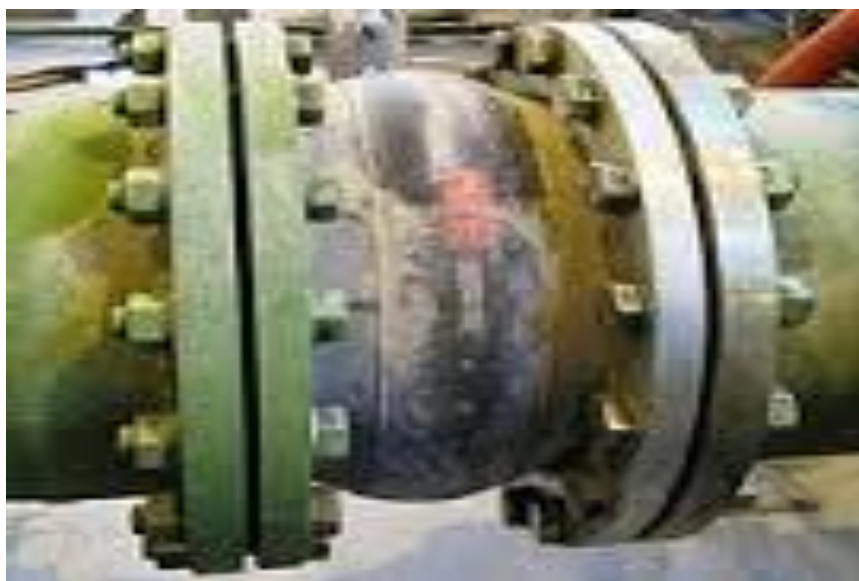
8.20 - rasm. Rezinali kompensator
