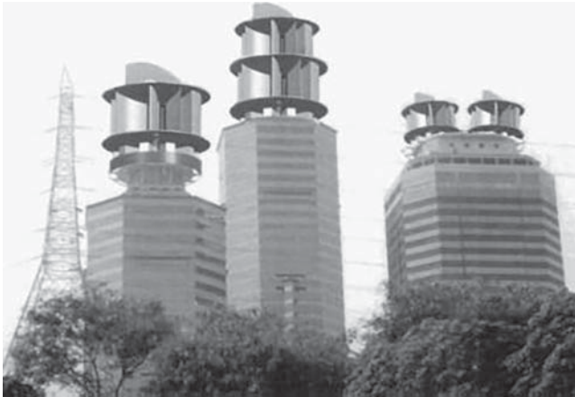
Figure 10.2 Integration of renewables in the building envelope. Source: Chong et al. [73]/with permission of Elsevier.
