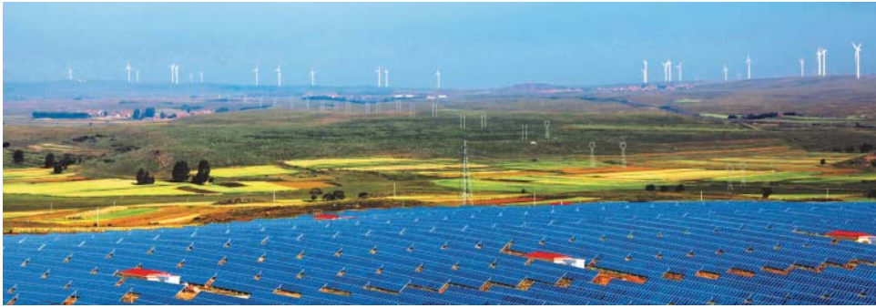
Figure 2.16 China's wind/PV/energy storage and transmission demonstration project. Picture source: SGCC.
