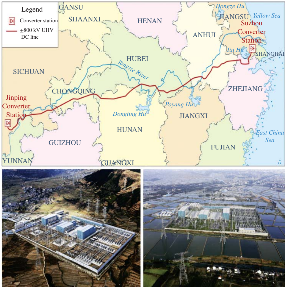
Figure 1.18 China's Jinping-Sunan ±800 kV UHV DC transmission line. Picture source: SGCC.
