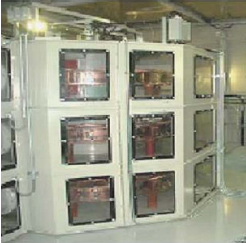
Figure A.9 Outside view of the collector ring of a VFT [5].
