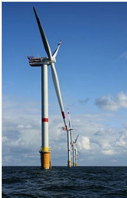
Offshore wind farm, using 5 MW turbines REpower 5M in the North Sea off the coast of Belgium .
