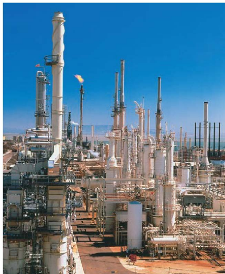
▲ Figure 25.9 Fractional distillation. Petroleum is separated into fractions by distillation and is subjected to catalytic cracking in a refinery, as shown here.
