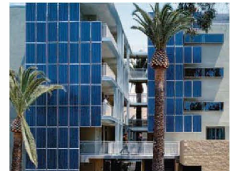
▲ Figure 12.13 Electricity from sunlight. Solar panels, made of silicon, are used both as an energy source and as architectural elements in this apartment building in southern California.
