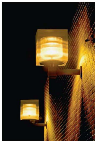
▲ Figure 7.27 Light from sodium. Sodium vapor lamps, which are used for commercial and highway lighting, have a yellow glow because of the emission from excited sodium atoms.
