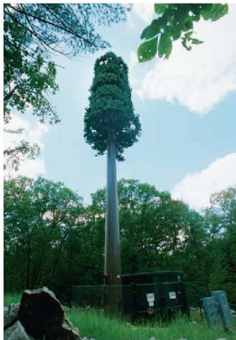
▲ Figure 12.21 Wireless communications tower. Towers like this (here, disguised as a tree) enable cell phone communication.
