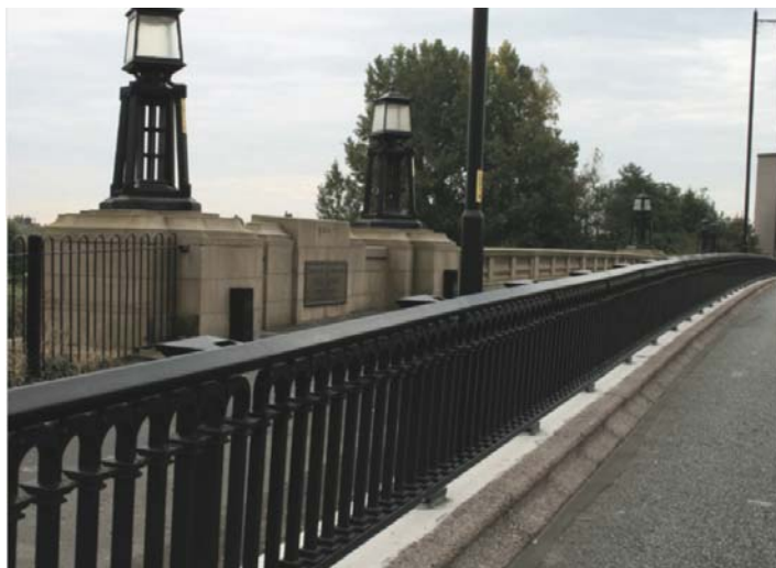
4.28-rasm. Ko‘prikka kiraverishda parapet
