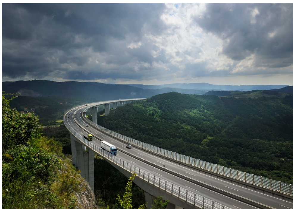
1.21-rasm. Murakkab estakada
