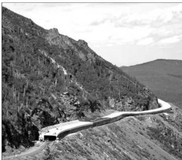
5.31-rasm. Chapda tosh to'kilishini oldini olish uchun yer usti yo'li, o'ngda ko'chkilarni oldini olish uchun sementbetonli himoyalash inshooti.
