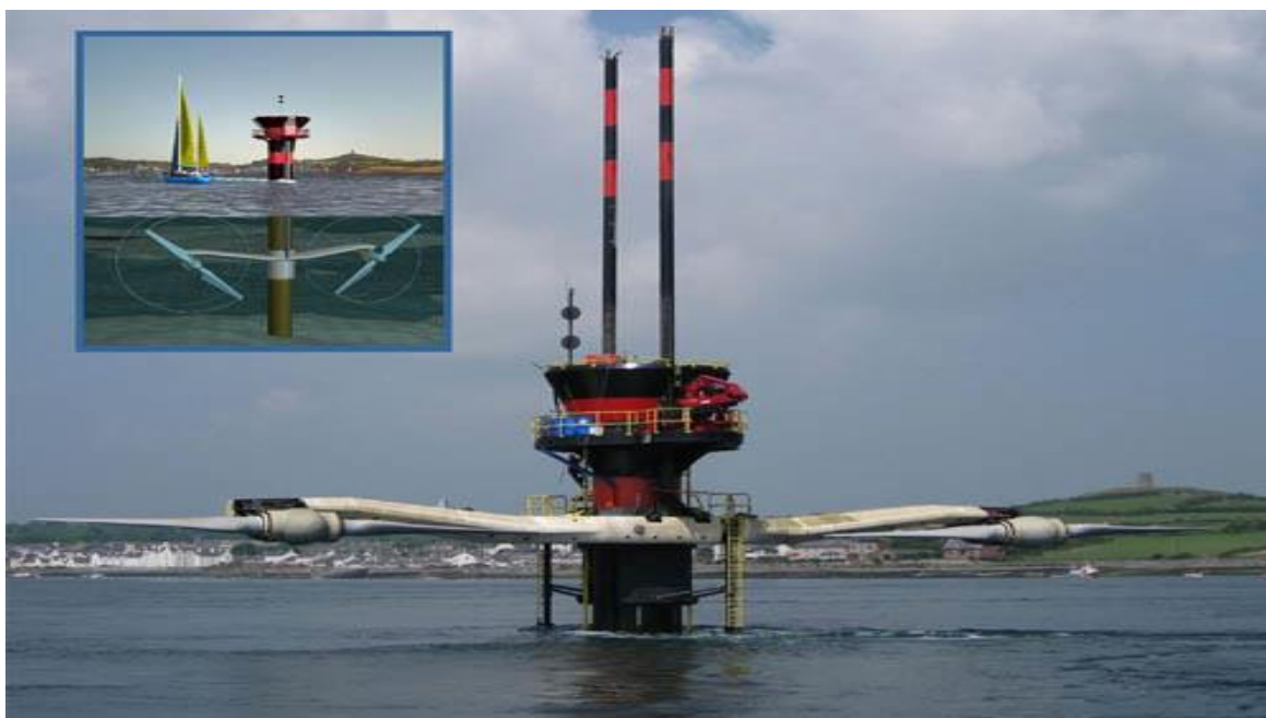
4.9-rasm. Suv sathning ko'tarilib tushish prinsipi asosida ishlaydigan eng katta turbina
