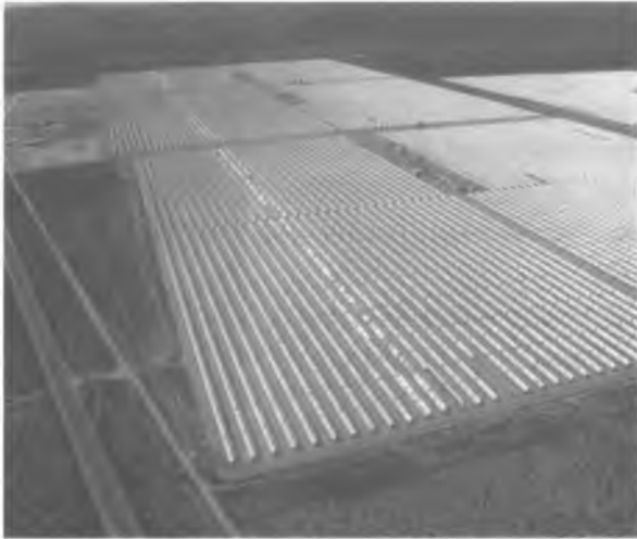
Figure 2.14. The world's largest-capacity solar thermal power plant, Solar Energy Generating Systems, is located in California, USA.
