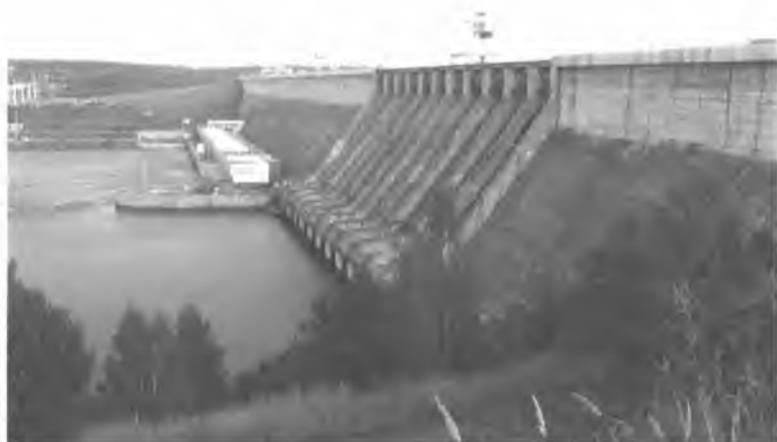
Figure 4.6. Top - Ilmsk HPP image.
