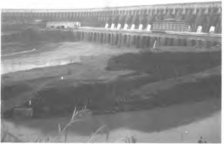
Figure 4.2. Image of Itaipu HPP.
