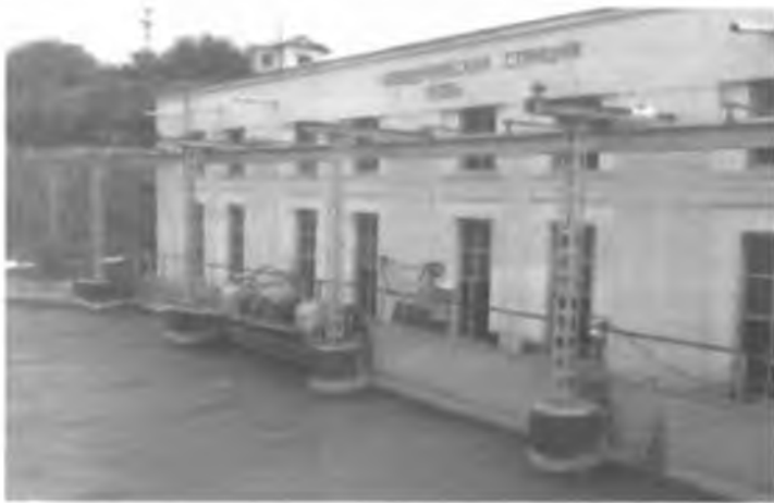
Figure 1.3. It was first built in Uzbekistan in May 1926 Bozsuv HPP.
