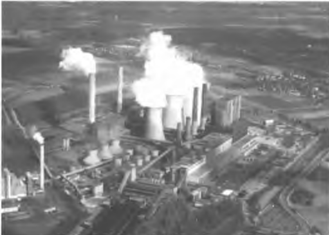
Figure 3.1. View of a thermal power plant.
