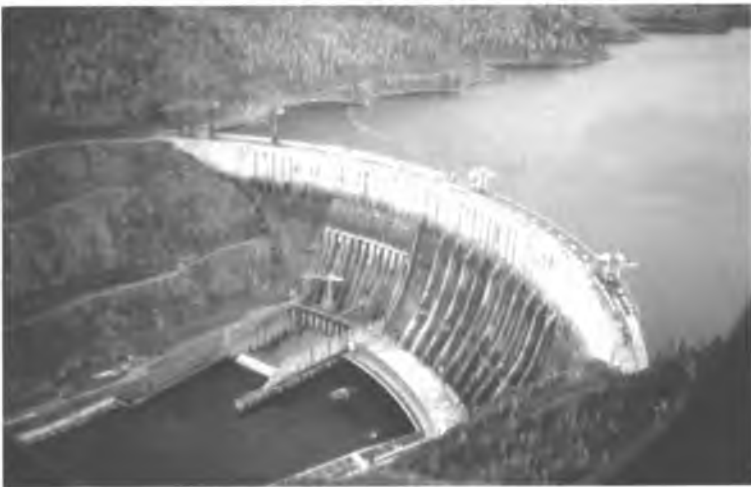
Figure 3.3. View of the hydroelectric power station.
