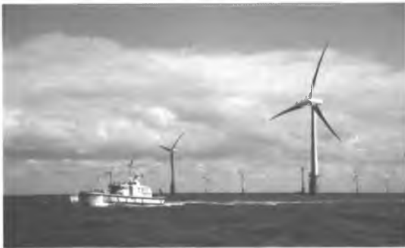
Figure 2.25. Thanet Wind Farm is the largest offshore wind park in the North Sea in Kent County, Southeast England.
