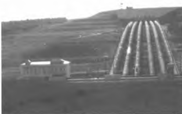
Figure 3.4. View of a hydroaccumulation power plant.
