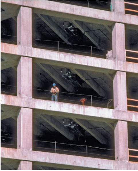
Photo 4.4 Reinforced concrete building frame.
