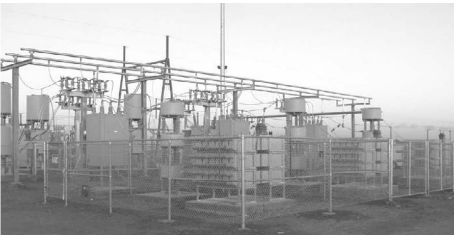
Figure 4-42. Static VAR compensator. Courtesy of Jeff Selman.
