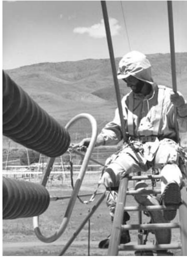
Figure 10-9. Bare-hand, live-line maintenance.
