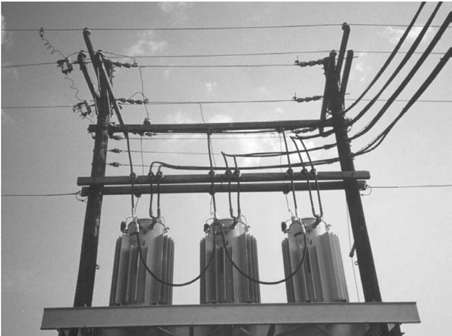
Figure 4-3. Transformer bank.
