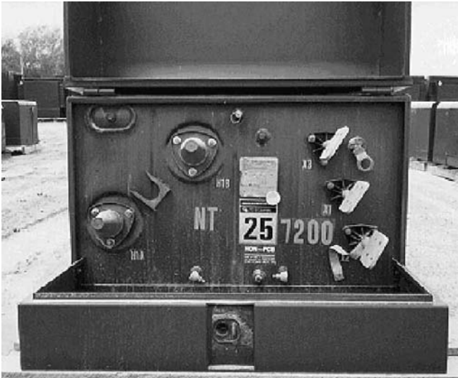
Figure 5-34. Switching transformer. Courtesy of Alliant Energy.
