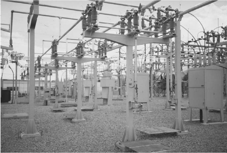
Figure 4-38. Examples of a typical electrical bus.
