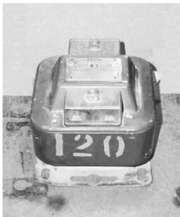
Figure 4-13. Low-voltage PT. Courtesy Alliant Energy.
