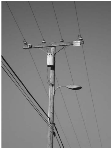
Figure 5-13. Transformer connections.
