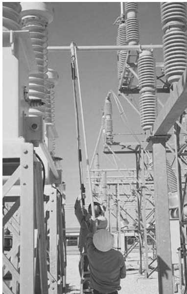
Figure 10-8. Live maintenance on transmission lines.
