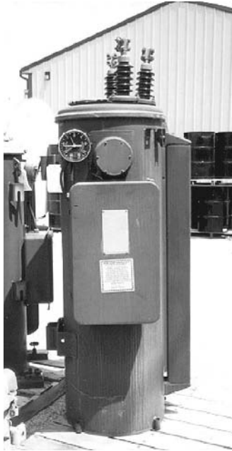
Figure 4-17. Single-phase regulator. Courtesy Alliant Energy.
