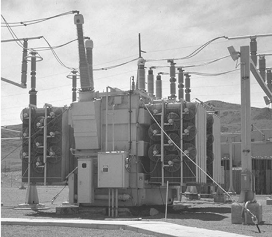
Figure 4-1. Step-down transformer.
