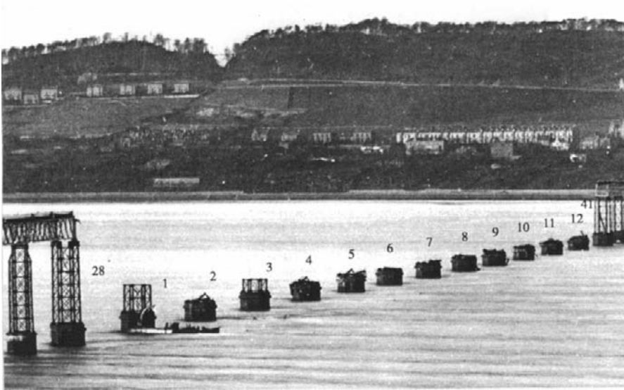
Fallen piers as seen from the south bank of the firth. For the purposes of the investigation, the piers between 28 and 41 were renumbered 1 to 12. (Courtesy of University of St. Andrews.)
