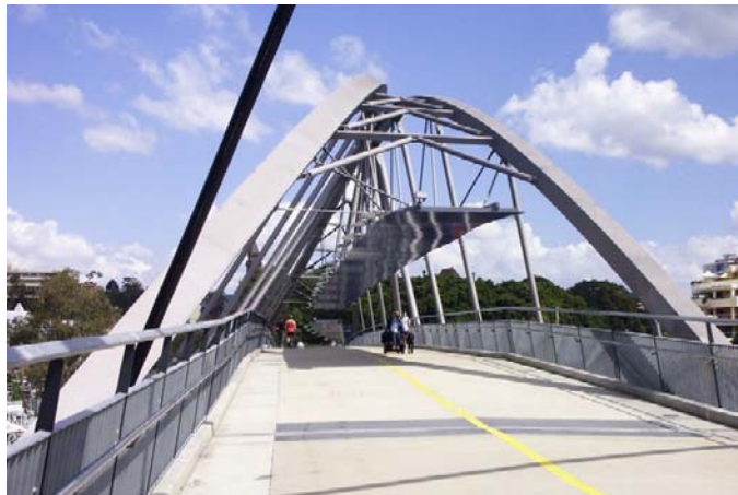
FIGURE 26.8 The Goodwill Bridge over the Brisbane River in Queensland, Australia. – 27 28 49.20 S 153 01 38.04 E
