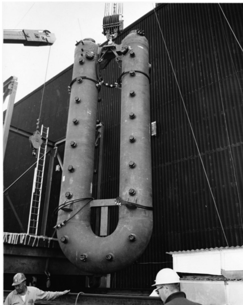
Figure 2.52 U-bend heat exchanger.
