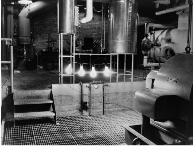
Figure 2.40 The first production of usable nuclear electricity occurred on December 20, 1951, when four light bulbs were lit with electricity generated from the EBR-1 reactor.
