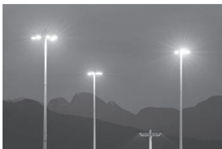
FIGURE 1.6 These high-temperature sodium vapor street lamps are made possible by use of a translucent \text{Al}_2\text{O}_3 cylinder for containing the sodium vapor. (David Nunuk / Photo Researchers, Inc.)
