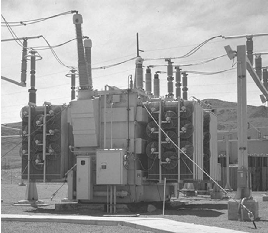
Figure 4-1. Step-down transformer.
