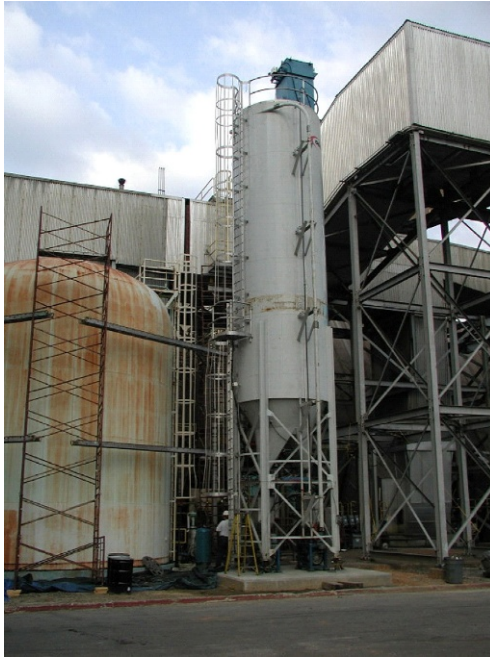
Fig. 3.9 Photograph of an ACI system, Showing the activated carbon storage silo (center of photo).
