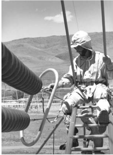
Figure 10-9. Bare-hand, live-line maintenance.
