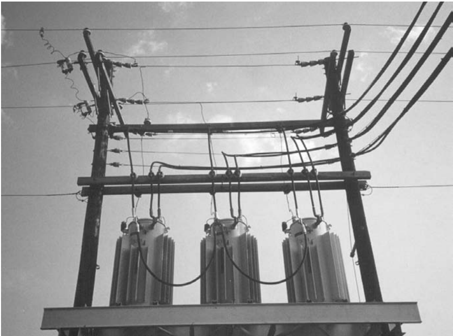
Figure 4-3. Transformer bank.
