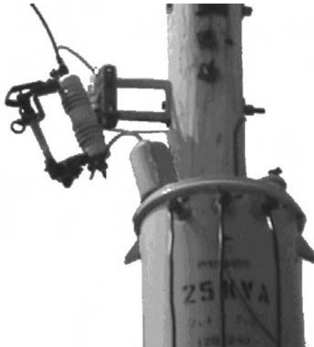
Figure 5.24. Distribution fuses.
