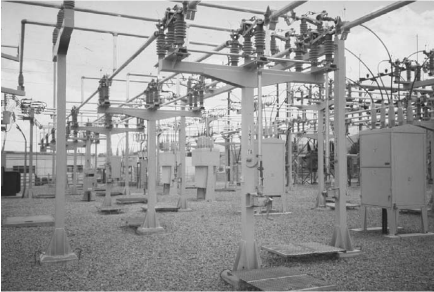
Figure 4-38. Examples of a typical electrical bus.
