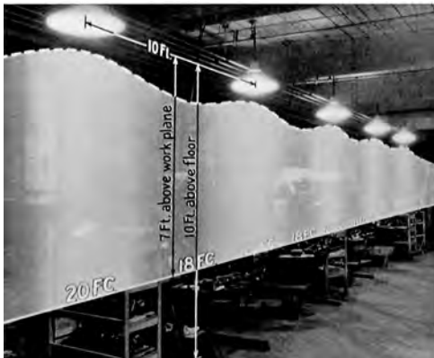
Too wide spacing results in poor distribution, as shown by the top illustration. For best seeing conditions, the illumination throughout the work area should be reasonably uniform. By properly spacing the outlets, as illustrated below, uniformity results.
