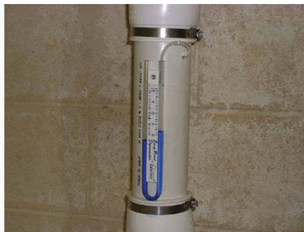
FIGURE 8.21 Measuring the pressure within a fluid using a manometer. The photo on the right shows a manometer used to measure the pressure difference in an exhaust system for radon within a basement.
