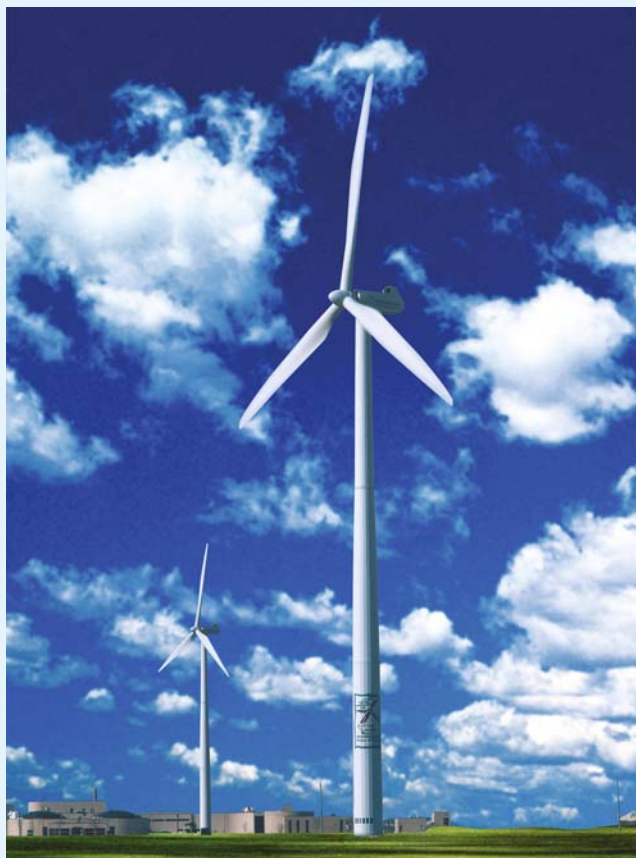
FIGURE 4.13 0.75 Megawatt generating windmills in Minnesota.
