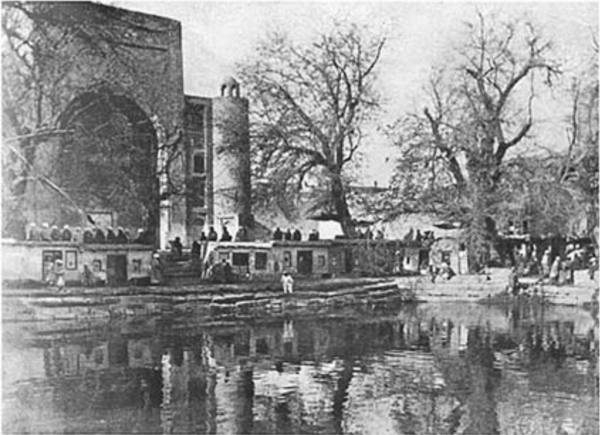
Main Reservoir, Bukhara
