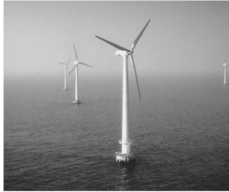
FIGURE 7.1 Vindeby offshore wind farm in Denmark. (From Vestas Wind Systems, Denmark. With permission.)
