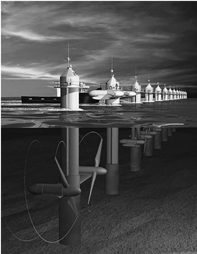
FIGURE 21.4 A proposed marine current tidal power system. (From Frankel, P., Marine Currents Turbine Ltd., Bristol, U.K. With permission.)
