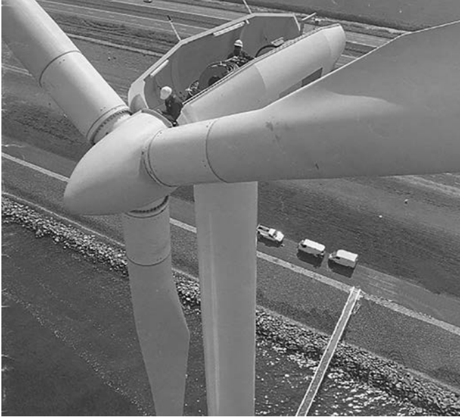
FIGURE 4.3 A large nacelle under installation. (From Nordtank Energy group, Denmark. With permission.)
