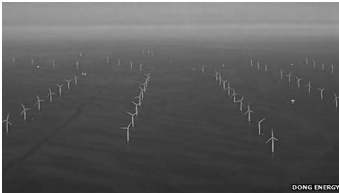
FIGURE 8.1 Walney wind farm. (From Dong Energy)
