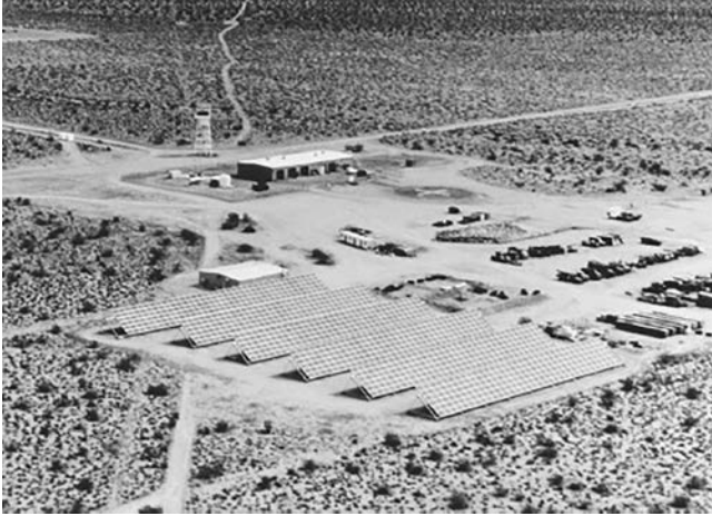
FIGURE 15.6 A 300-kW PV–diesel hybrid system in Superior Valley, California. (From ASE Americas, Inc., Billerica, MA. With permission.)
